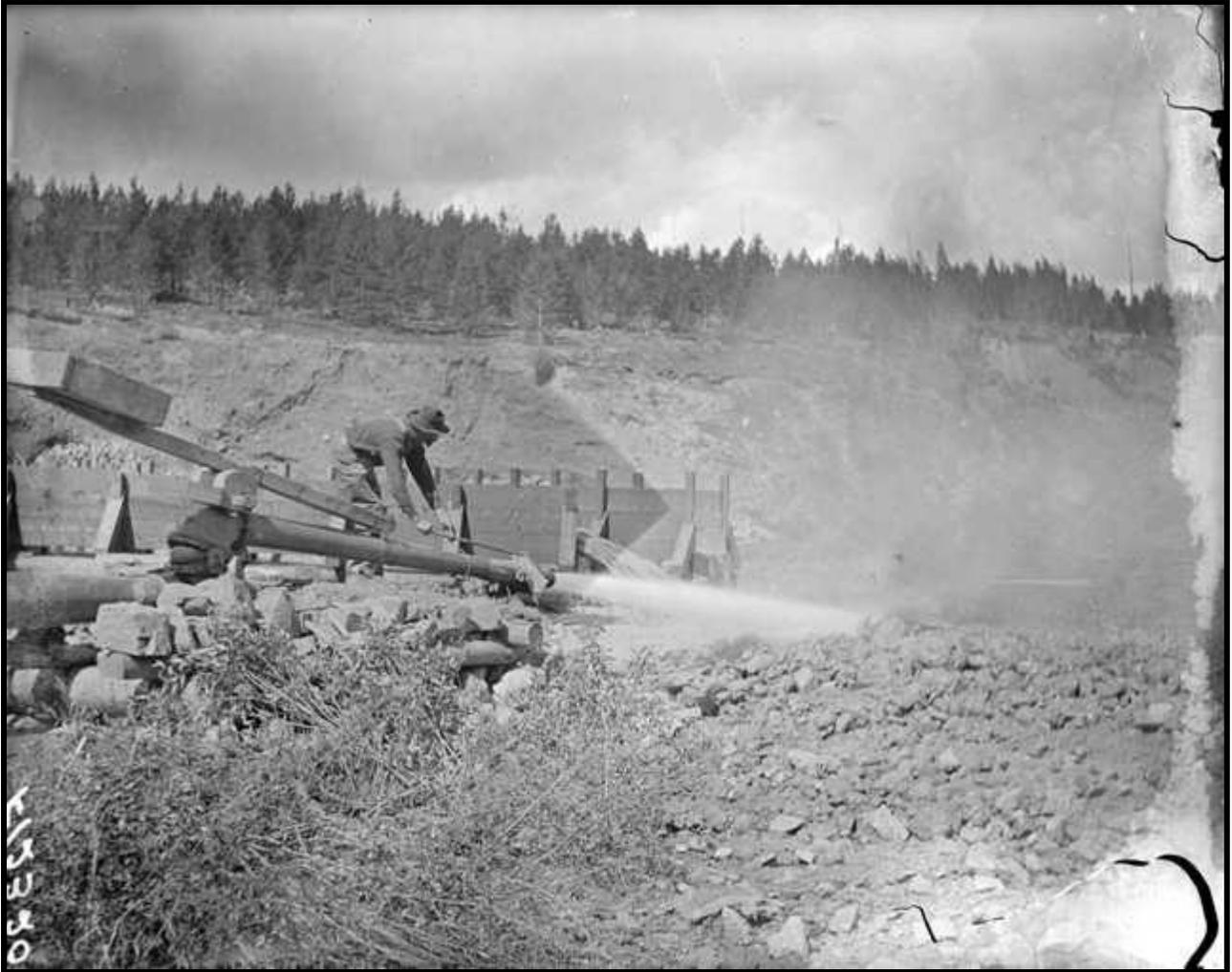
Figure 2.41: In this 1880s northwestern view, a worker uses a hydraulic monitor to push gold-bearing gravel through sluices on the Peabody Placer. The box extending left from the monitor was a counterweight filled with cobbles. Source: Denver Public Library, X-60107.
