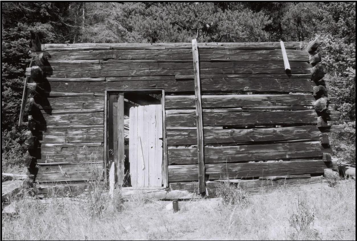
Figure 2.72: The boardinghouse is a sound example of workers' housing erected at large placer mines in Colorado. The walls were carefully constructed with hewn logs and nested chinking to present smooth surfaces. Source: Author.
