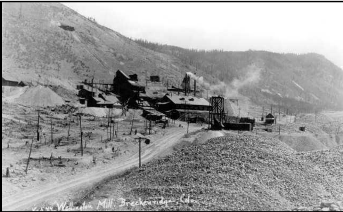
Figure 2.5: View east of the Wellington around 1912, shortly after a roasting and concentration plant, center, were added to the mill, left of center. Source: Denver Public Library, X-61039.
