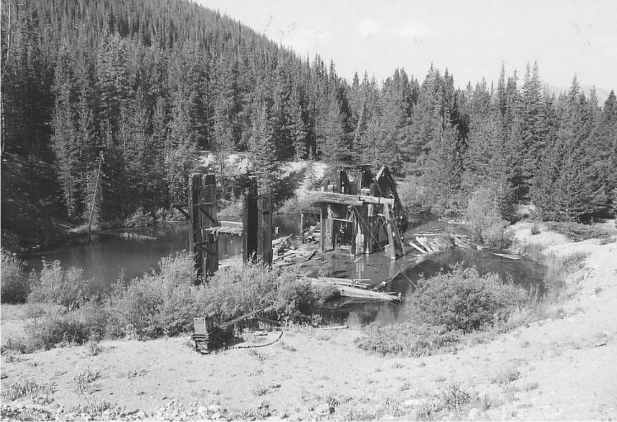
Figure 2.24: The rear quarter view depicts the Reiling Dredge hull in upper French Gulch, which was the last point of operation. The two posts left of center held the tailings stacker, and the bucket-line extended outward from the hull's far end. The hardware and superstructure have been dismantled. Overall, the site retains a high degree of integrity and includes the archaeological remnants of a base camp, out of view to the left. Source: Author.
