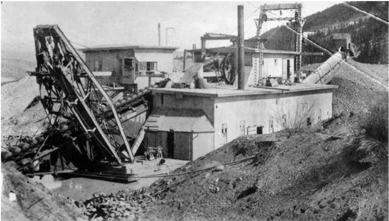
Figure 2.23: The photo depicts the Reiling Dredge near the mouth of French Gulch around 1909. Note the dredge's closed-connected bucket-line at left. In the cabin at upper left, a worker operated winches that elevated the bucket-line and tailings stacker, and adjusted the mooring lines. Source: Denver Public Library, X-60158.
